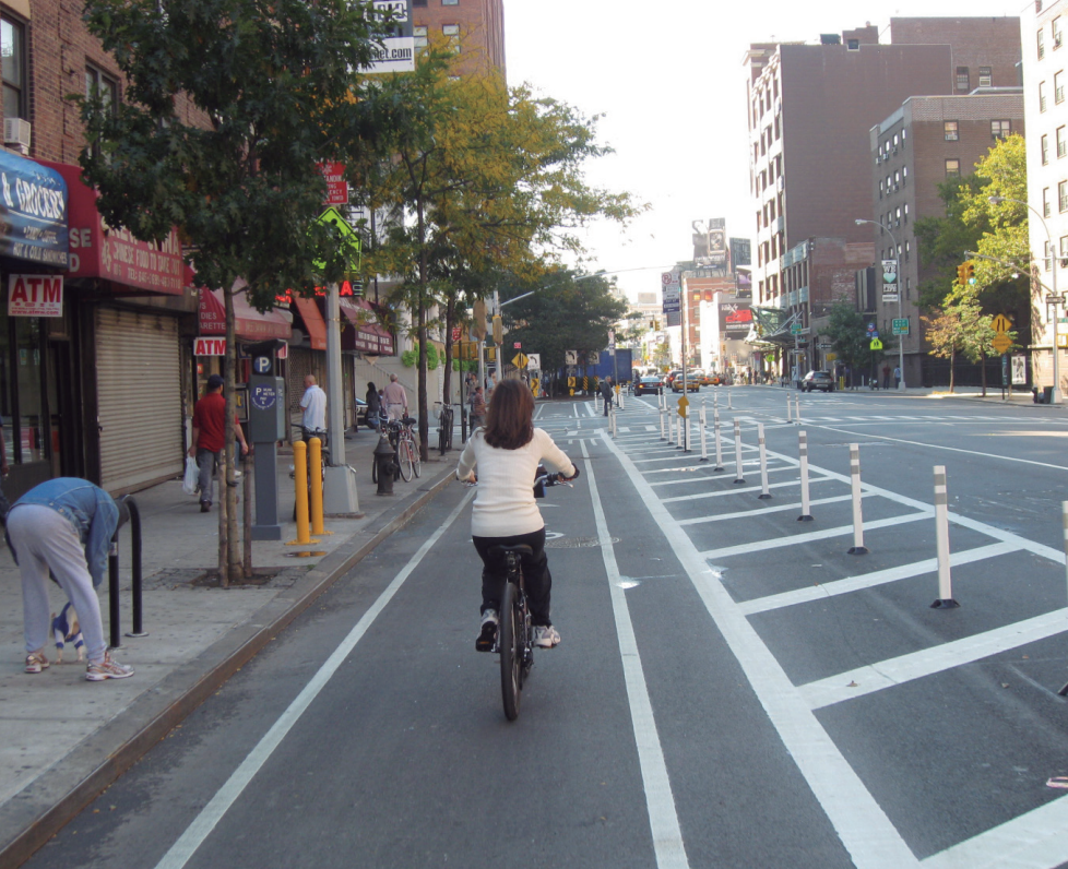
Protected bike-ways in New York, USA. A painted line on the pavement is not safe enough; it needs a physical separation like the one shown in the photo.
