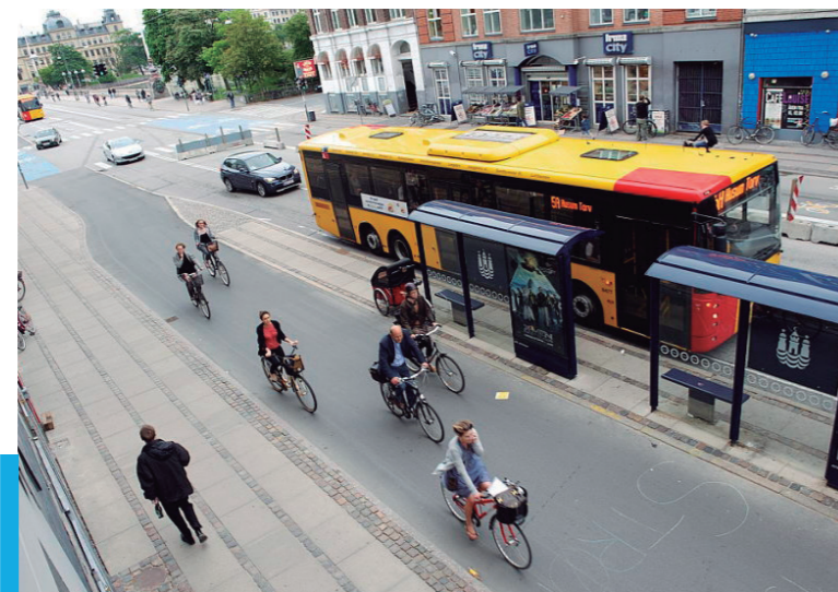
Approach road Nørrebrogade after rebuilding - note how wide the pavement and cycle track are.
