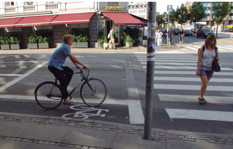
Safe and secure intersections in Copenhagen also allow easy passage for cyclists. This design shown uses a 1.5m wide cycle lane while another design takes the cycle track right to the stopline.
