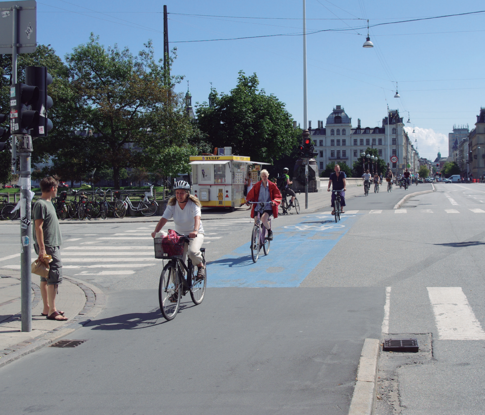
Nørrebrogade second generation cycle tracks (3-4m wide) established in 2011 and 12. As the blue cycle crossing indicates, the cycle tracks have been widened from the first generation standard of 2 m up to the present 3-4 m.
